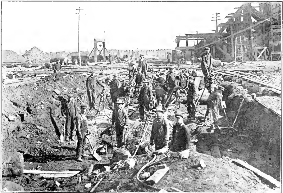
Fig. 66—Commencement of No. 3 shaft, 5 compartments, Creighton mine, 1915.
